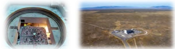
**Fig. 1.** The Idaho National Laboratory's Transient Reactor Test (TREAT) Reactor. (Left) View of 19x19 array of driver fuel assemblies. An irradiation test vehicle is visible at the center position of the core. (Right) Ariel view of the TREAT facility at the Idaho National Laboratory Materials and Fuels Complex.
